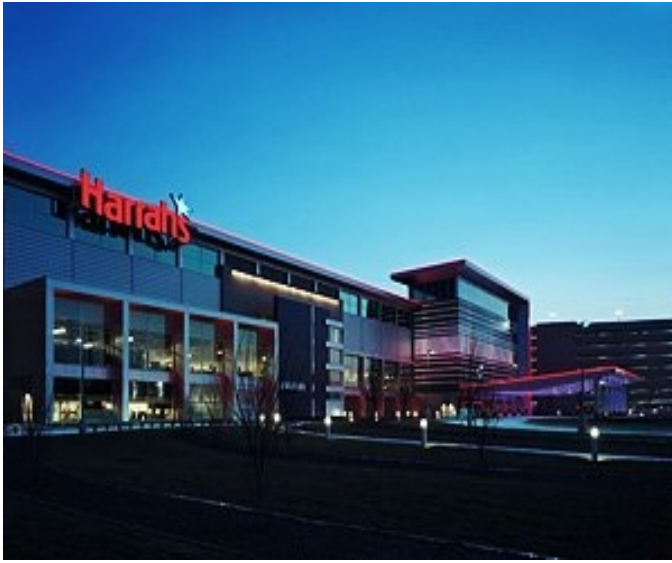
Maintenance work at Harrah's
